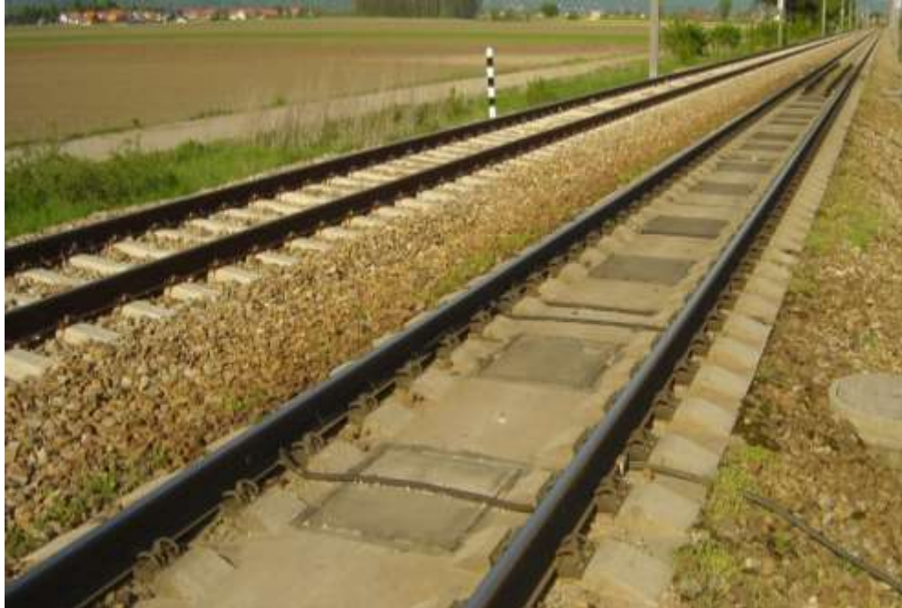
Langenlebern - First Installation PORR Slab Track System in 1989
