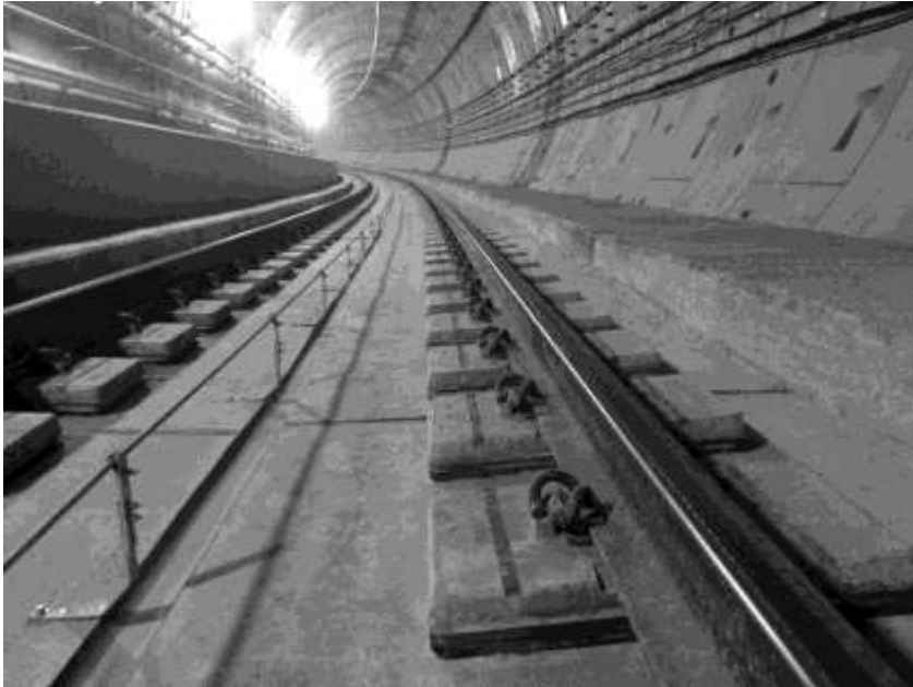
LVT System with e-clip fastening system
