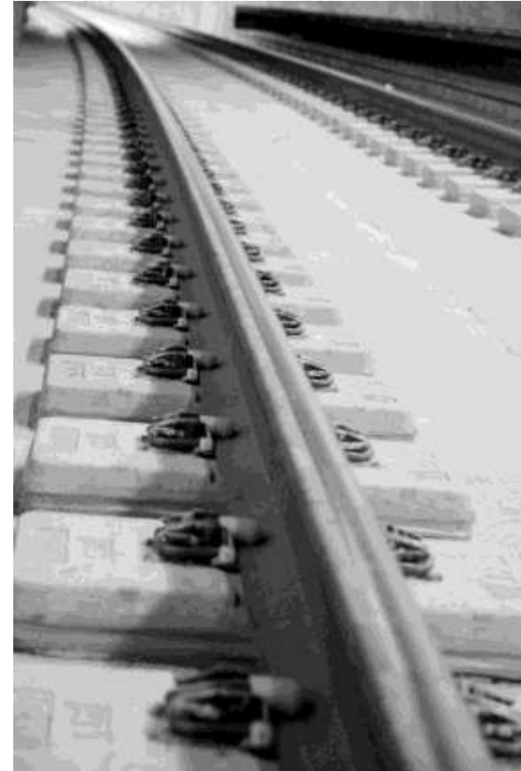
LVT System with Fastclip fastening system
