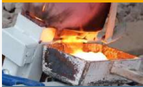
Aluminothermic Welding
