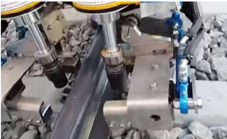
SKL-14 Installed with Robel SKL Clipping Machine
