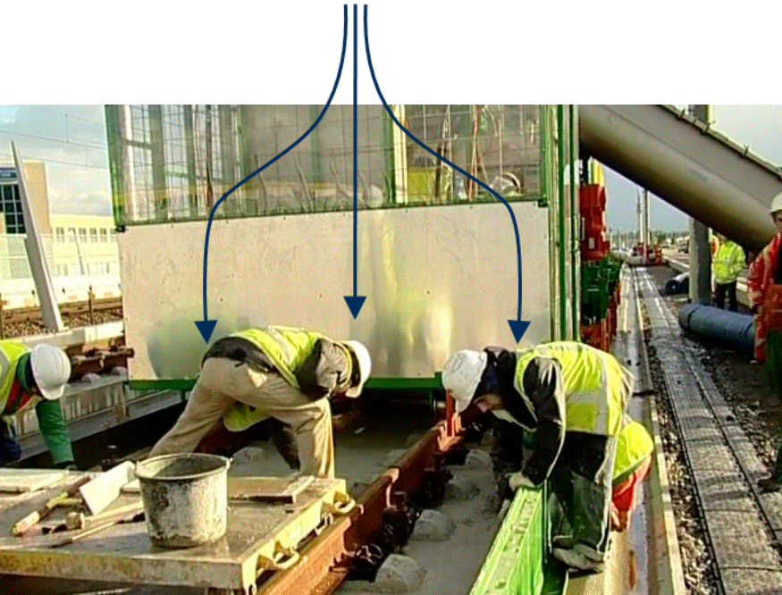
Concrete casting platform
