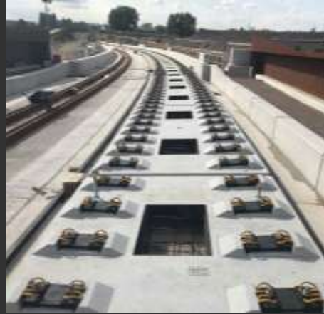
Slabs with low toe-load fasteners for bridges (lengths varied)
