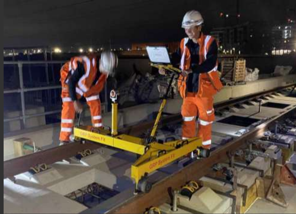
And sometimes by night (hogging of steel girder spans)
