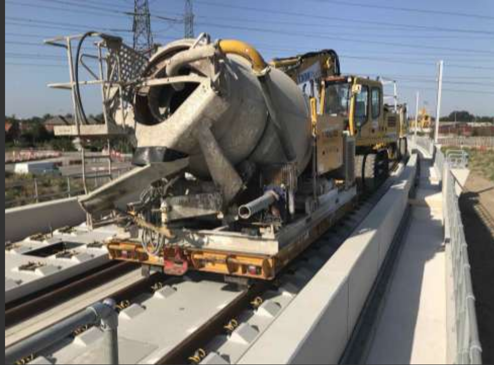
Concrete was delivered mostly direct by crane Not possible everywhere!
