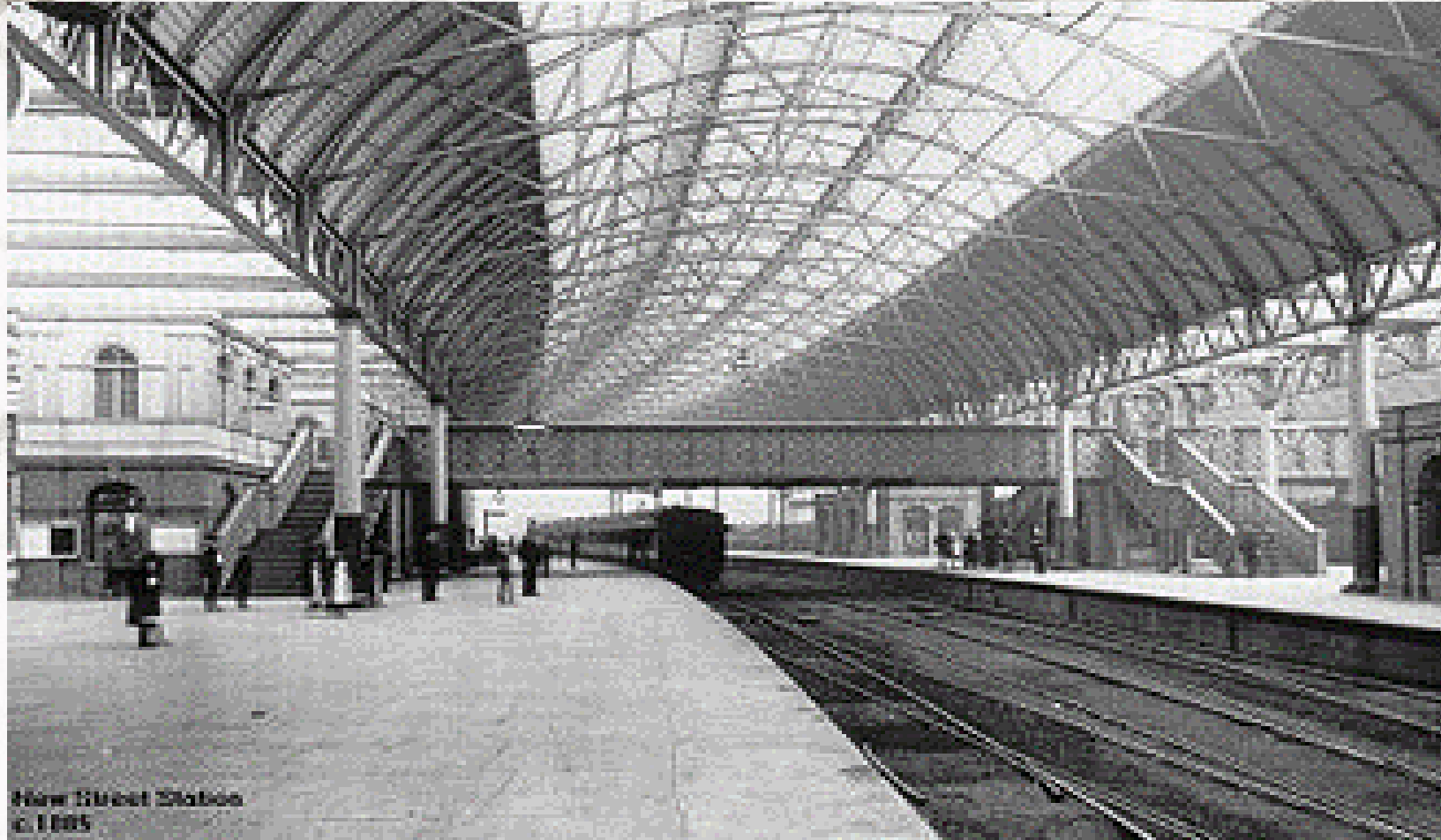
Midland Railway's extension of New Street station, in 1885
