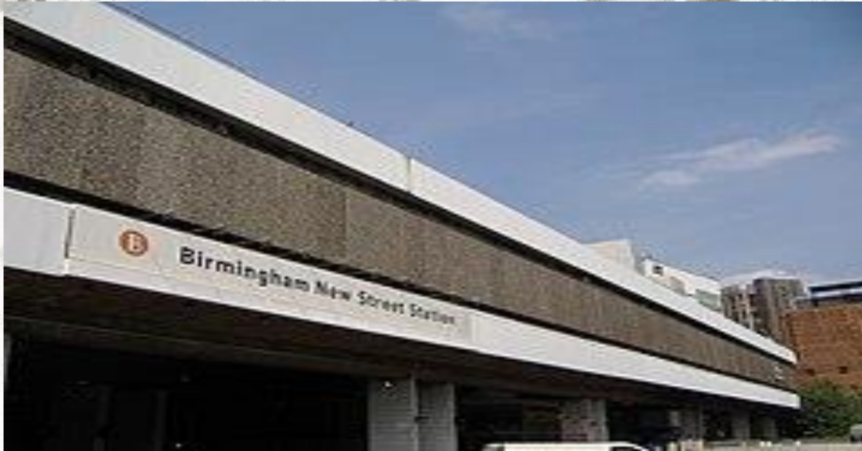
The concrete external architecture of the 1960s station
