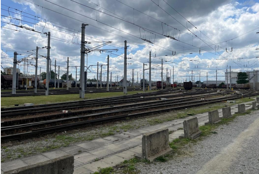
Marshalling yard Graz, Austria
